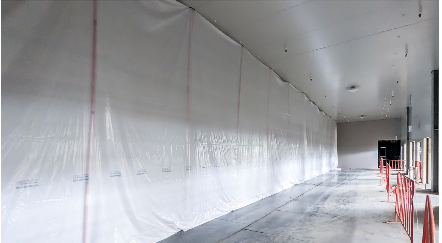
ZipWall® installation in process.
