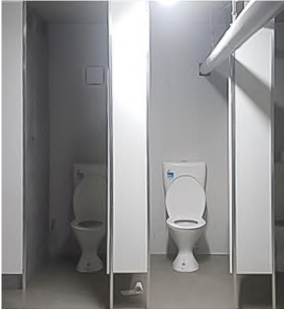
FastWall used to create onsite toilet cubicles.
