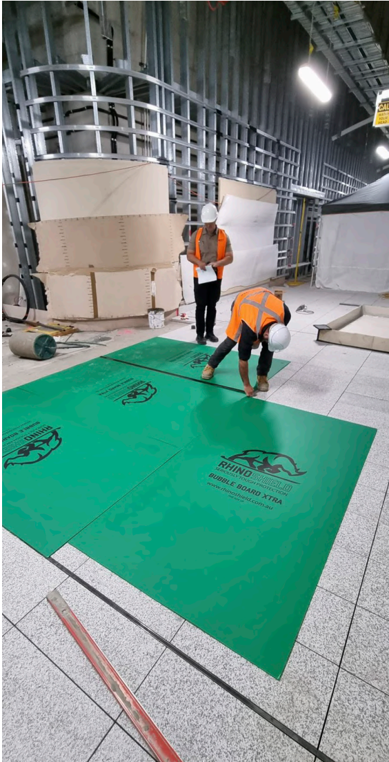
Bubble Board Xtra protecting premium granite pavers. Image Source: NSW Government
