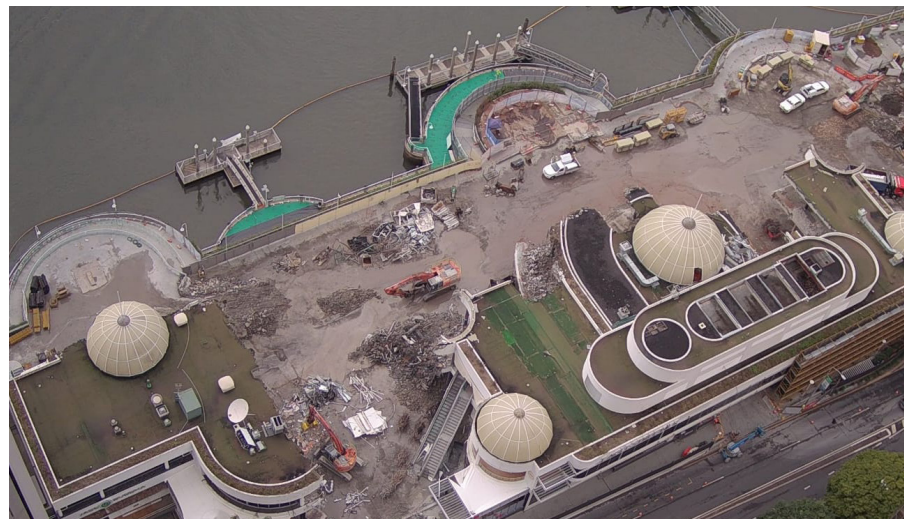
The Eagle Street Pier site set for demolition.
